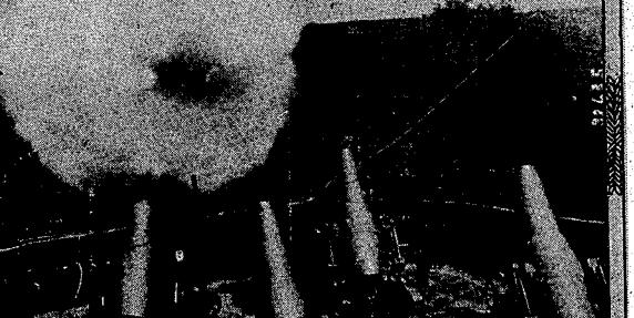
Battery of 12-inch mortars, part of the protection of New York harbor. Recently these mortars were tested, and were successful in hitting targets 12 miles away. They are fired through electrical connections.
