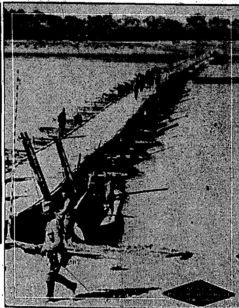
Pontoon bridge constructed across a river following the blowing up of the highway bridge by retreating forces.
