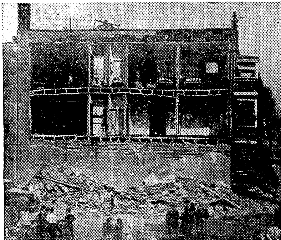
The occupants of two flats in Montreal miraculously escaped death or serious injury when the side wall of the dwellings crashed into a vacant lot. The photograph shows the scene shortly after the crash. The occupants of the lower flat, forewarned, moved furniture to opposite side of the building as may be noted in the picture.
