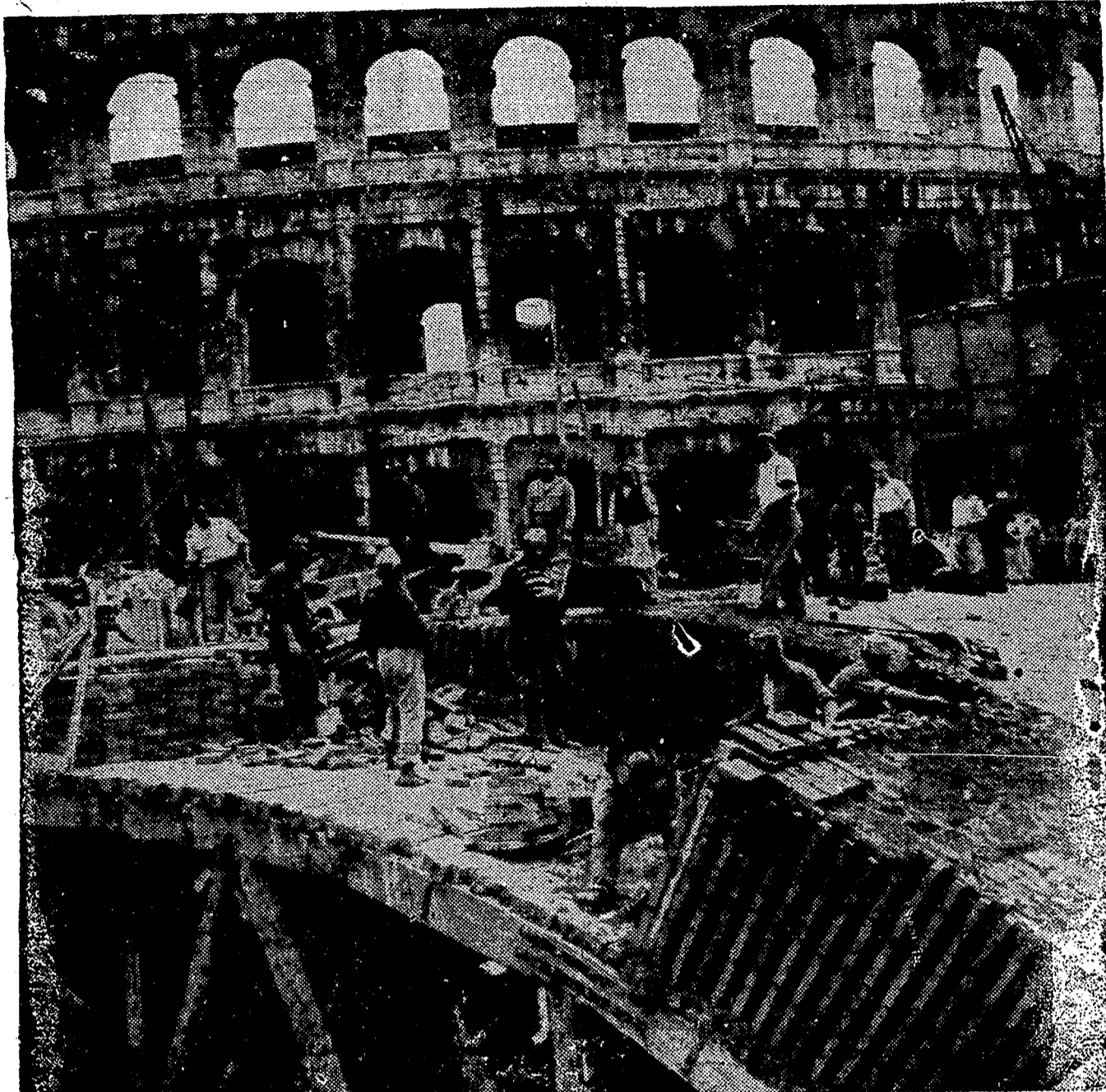
The ancient Colosseum in Rome, Italy, provides an interesting backdrop for these bricklayers as they construct the roof of a subway in the Eternal City. The "Metroolitana," as the subway is called, is designed to run from the central railway terminal in Rome, beneath the Esquiline and Quirinal hills to Piazza Venezia, to the Colosseum and then to St. Paul's Gate, where it will emerge from its tunnel and connect with the existing surface electric railway line to Ostia on the Tyrrhenian Sea.
