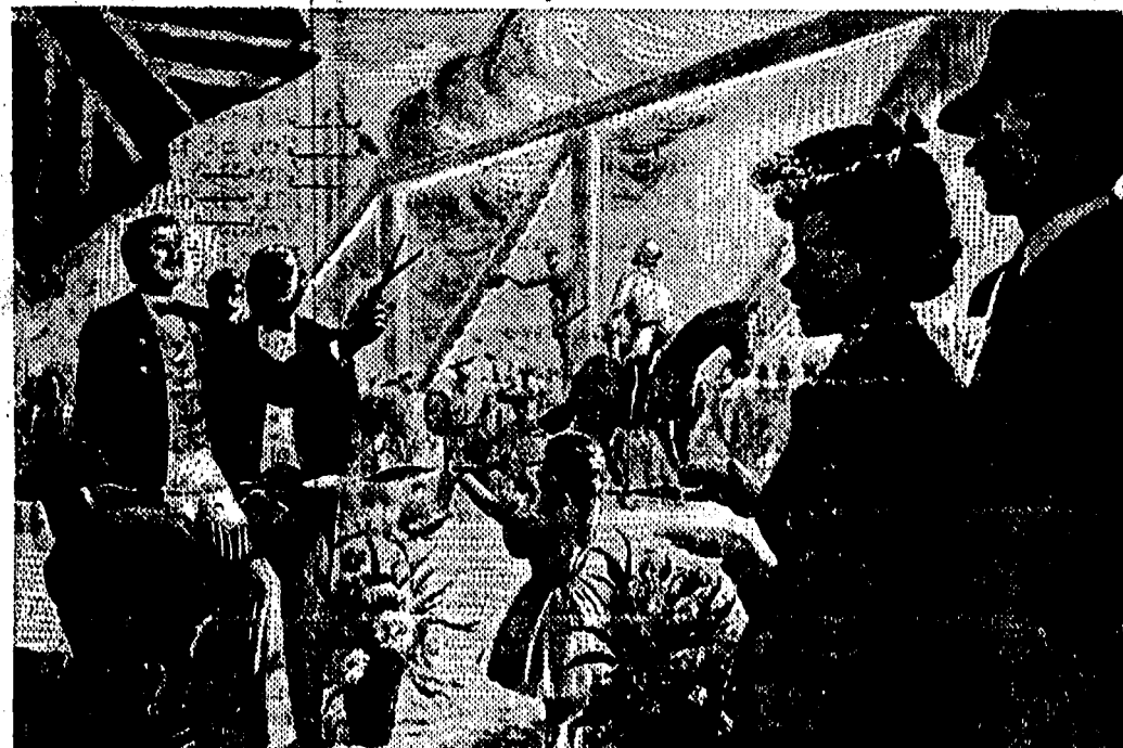
On July 23, 1904, Sir Henry Joly de Lotbiniere opened the Fraser River Bridge—the first bridge to span the mouth of the Fraser and provide a direct rail and road link to the United States.
