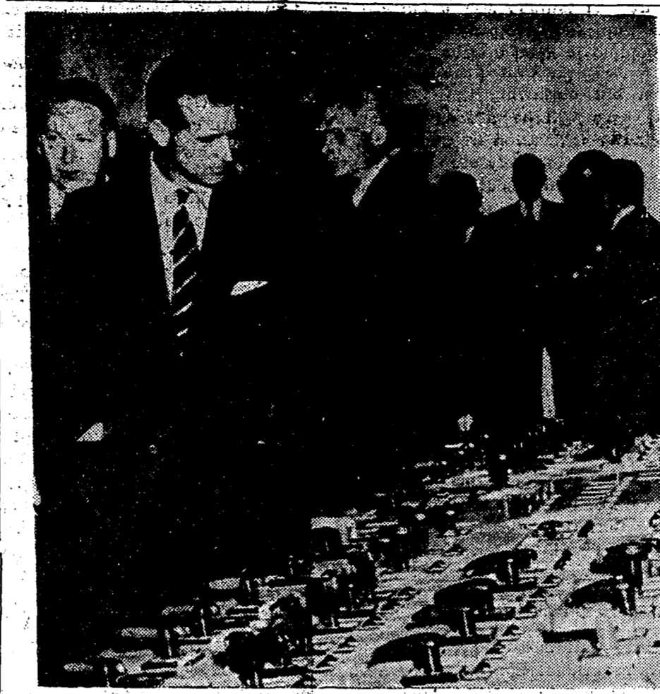
At Kemano, B.C., Prince Philip pauses long enough to show bewilderment at the array of dials on a control panel of the newly constructed power station there. He displayed considerable technical knowledge as he toured the Kitimat and Kemano plants, but showed no desire to toy with the controls of the biggest power development in the world built by private enterprise.
