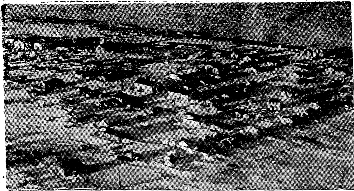
Aklavik, the Canadian town on the edge of the Arctic ocean, is in danger of sinking into the perma frost, moss and mud on which the town rests. On the present townsite it is impossible to build roads, sewers or solid substantial buildings, and, as the town grows, danger of epidemic is always present. So the town is being moved, but many who know the far north wonder where a suitable site can be found within hundreds of miles.
