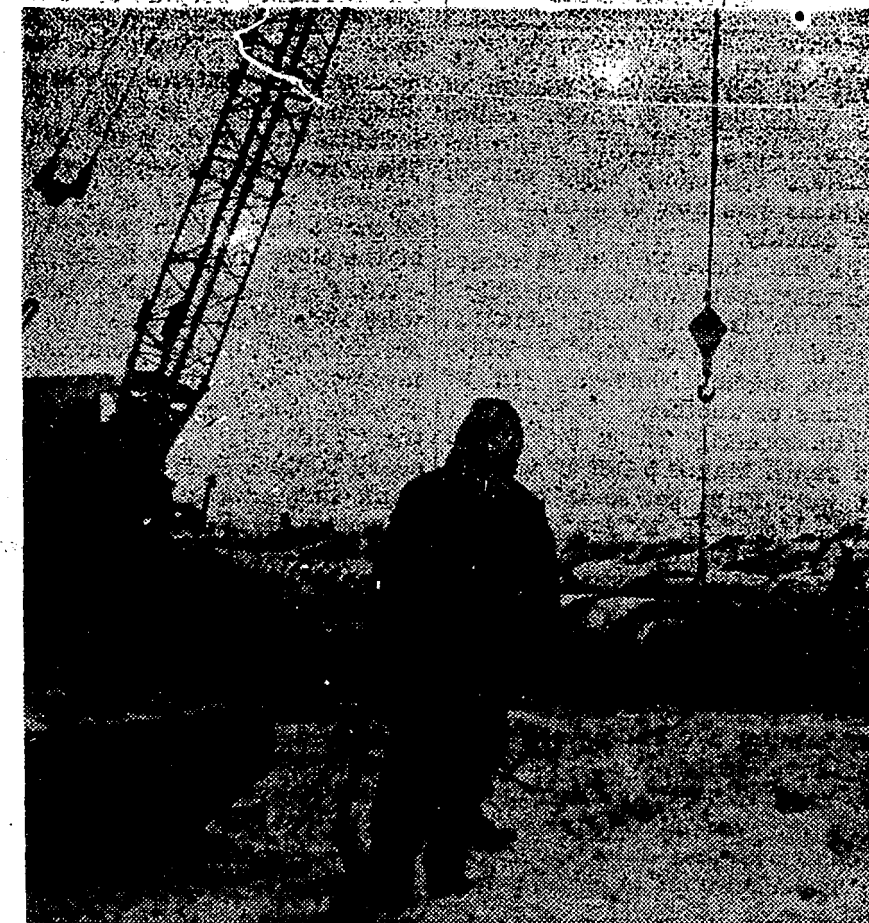
Away she goes! Two hundred and seventy-five tons of 34-inch pipe, coating and concrete river weights are shown here sliding into the Assiniboine river near Portage la Prairie, Manitoba. The pull was made by five tractors, with an assist at the river's edge from a drag-line and derrick. With the river section in place, couplings can be made on either side and the pipeline continues on to the next obstacle.
