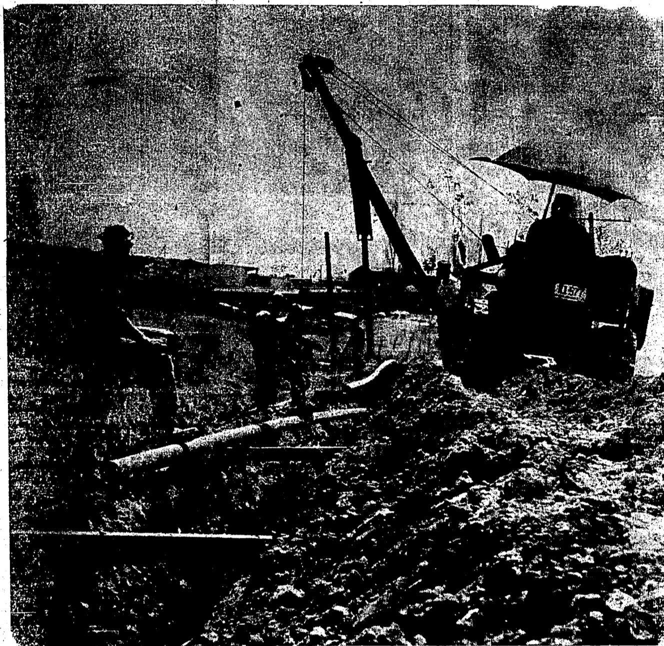
NATURAL GAS isn't here yet, but concrete evidence of its coming is on view in Summerland where this week contractors Dutton-Williams started work on laying the pipe line into Summerland for the Inland Natural Gas Co. Ltd. The above picture shows pipelayers at work along the KVR road, under the shadow of Giant's Head.
