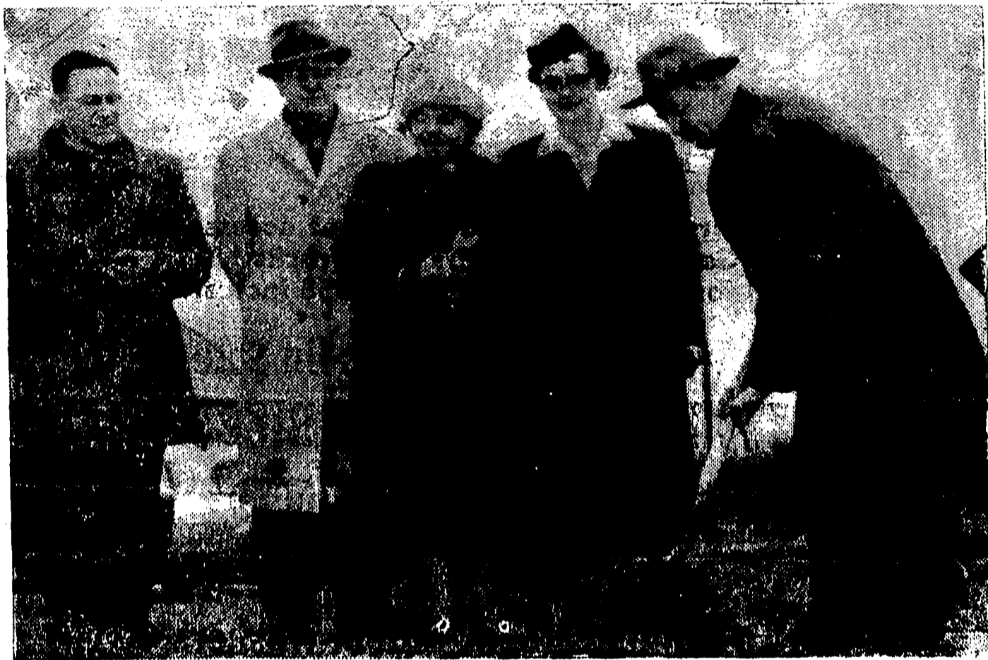
Reeve Atkinson turns the first sod to launch construction of Summerland's Health Centre and library building.
