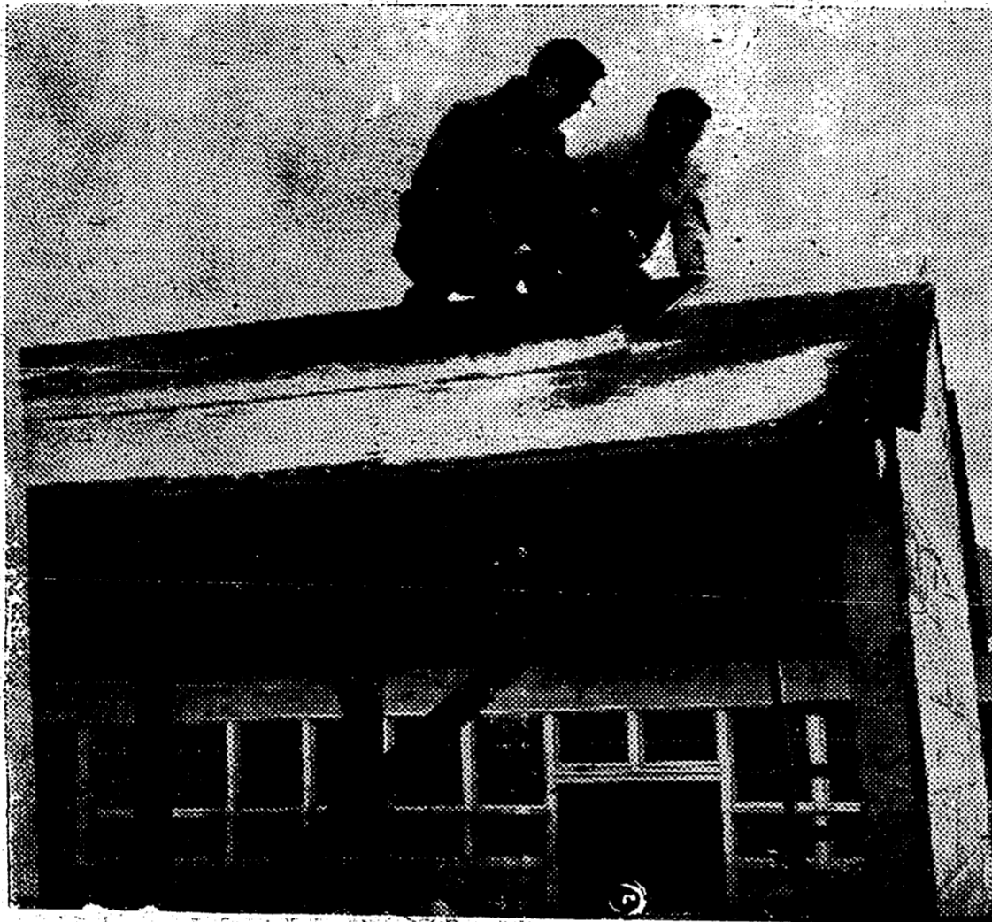
Working on the Key Club bicycle shed
