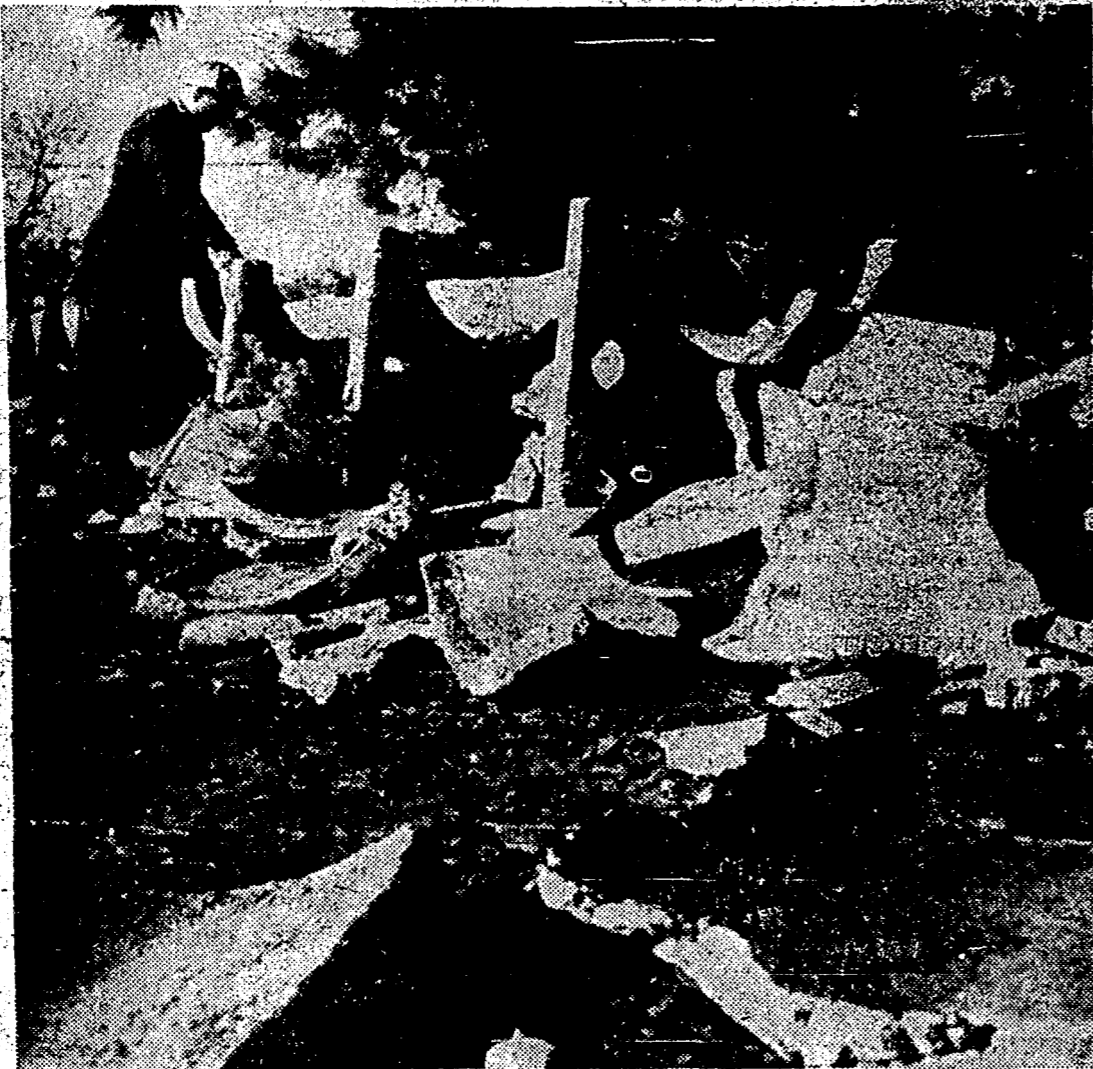
George Geres of the municipal crew, inspects damage caused recently by vandals to the irrigation flume in Garnett Valley. The municipality is offering a $50 reward for information leading to those causing the damage, which is estimated at $300.
