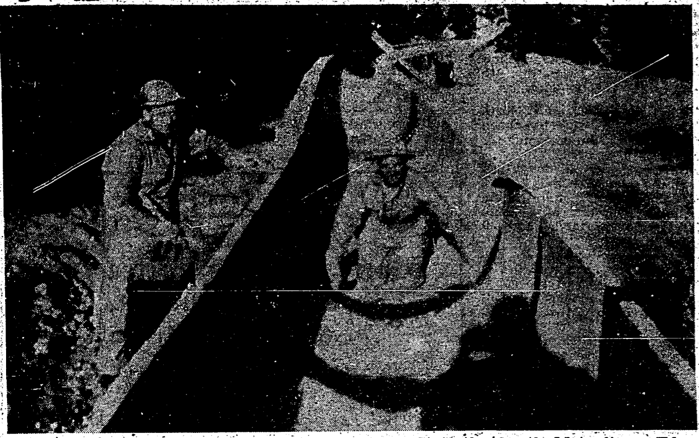
NEARING END OF LINE flume. It is the South Main line. The Joe Van Gammeren, left, and Frank Lauer are putting the finishing touches to the newly installed pre-cast irrigation flume was pre-cast in the municipal shops in Summerland.
