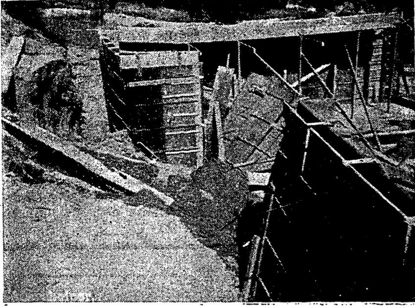
A Smith & Hill cement mixer driven by Joe Maddison backed up to pour the foundation and the dirt gave way and mixer, truck and all slid down into the excavation as shown above. Note the spilled cement which is darker than the dirt fill. The other picture shows the mixer as Bud's Service is towing it out inch by inch. They had to cut it away from the truck. Equipment damage will amount to about $500. The frame was twisted on the truck. The truck had stopped about 9 feet from the cement forms. An adequate distance, it was thought.
