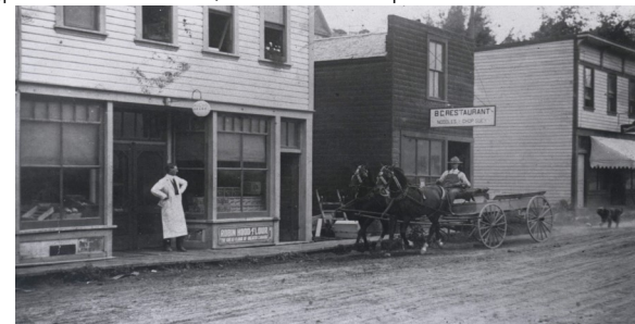
Businesses on Lakeshore Drive South
