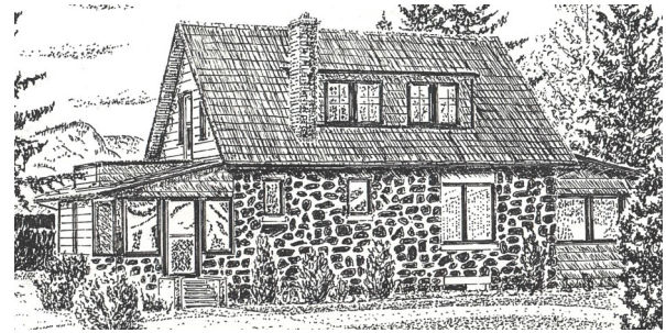
3. Bowering Home (1912) (10515 Quinpool Rd) This stone, end-gabled cottage is another example of the Arts & Crafts Movement in Summerland. It was built for the Jabez Bowering family by John Gordon Robertson and Alfredo Biagioni using local fieldstone which was excavated when digging the basement. It was one of first homes in town to have hot water heating. Jabez, a retired minister from Manitoba, was the postmaster in West Summerland for thirty years. Due to his health, the family left the home in 1939 to a new post office on Main Street with living quarters in the rear.
